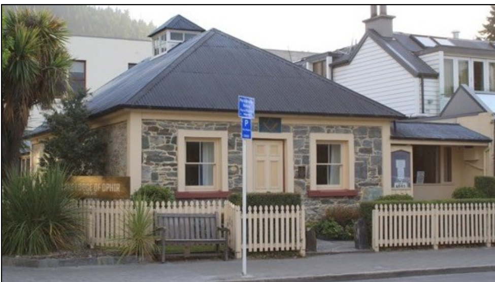
After the restoration project in 2008
